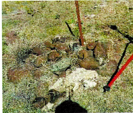
Photo of the galvanized pipe monument, firmly set flush with the top of a mound of stone, 3 1/2 ft. base, 1 ft. high.
