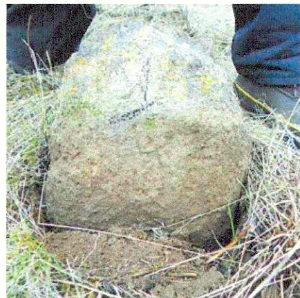
What appears to be a double image, is actually the 1/4 markings of both Henderson in 1881 and Wilkes in 1917.
