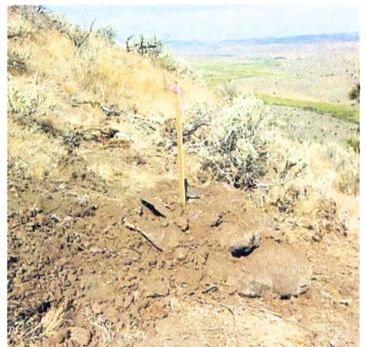
Set brass cap monument to within 8" of the surface in a mound of stone 3 feet at base around monument. Original stone is buried on the West side of monument.
