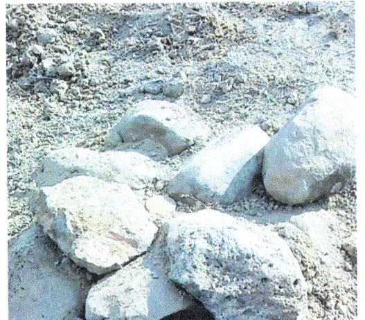
Set brass cap monument to within 8" of the surface in a mound of stone 3 feet at base around monument. Original stone is buried on the West side of monument.
