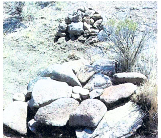
Set brass cap monument to within 8" of the surface in a mound of stone 3 feet at base around monument. Original stone is buried on the north side of monument. Note the mound of small stone I placed 3.5 feet East of the monument being residue from digging the monument hole.
