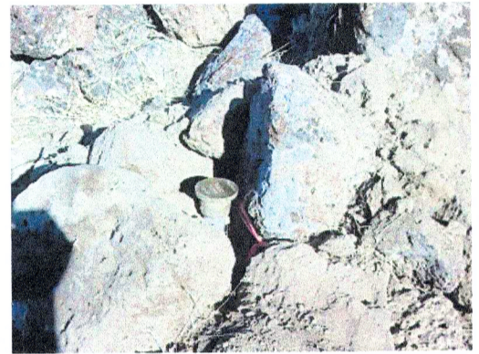
Set brass cap monument to within 8" of the surface in a mound of stone 3 feet at base around monument, original stone is buried on the North side of monument.
