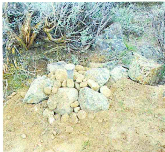
Brass cap and mound of stone as they appeared before covering the mound with soil to assist in protecting and stabilizing the mound. I then reset the steel fence post alongside the mound to aid in locating the monument.
