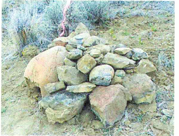
Buried the monument to within 10 inches of the surface. Original stone was placed upside down and placed on the North side of the Brass Cap. I placed a large mound of stone around the brass cap monument.
