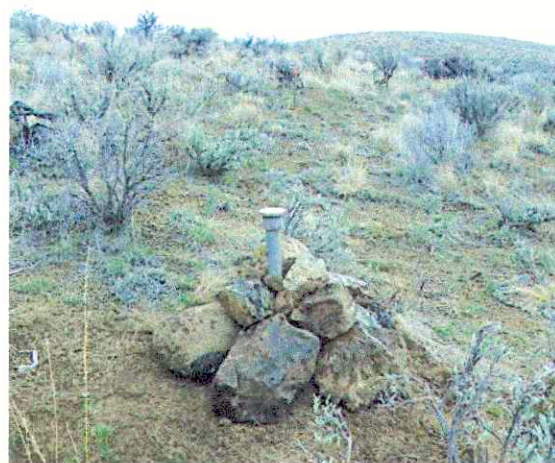
Buried the monument to within 10 inches of the surface. Original stone was placed upside down and placed on the West side of the Brass Cap. The remains of the original mound of stone was then placed around the Brass Cap. Notice the reference pin located in the background near the top center of photo.
