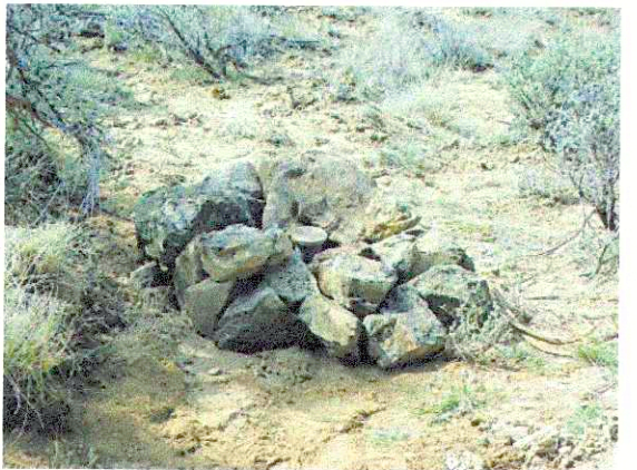
Brass cap and mound of stone as they appeared before covering the mound with soil to assist in protecting and stabilizing the mound.
