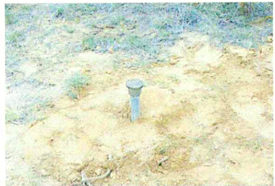
Buried monument to within 8 inches of the surface. Original stone was placed upside down with the tip above the surface on the North side of the Brass Cap. Using the only stone available in the general area I placed a very small mound around the monument. There are no other stone available in the general area of the monument.
