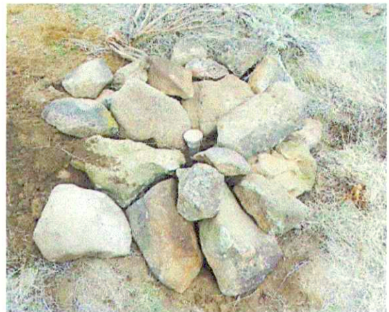
Brass cap and mound of stone as they appeared before covering the mound with soil to assist in protecting and stabilizing the mound.
