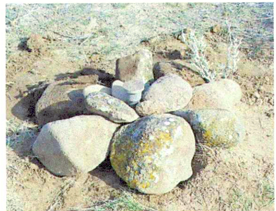
Brass cap and mound of stone as they appeared before covering the mound with soil to assist in protecting and stabilizing the mound. I then reset the steel fence post alongside the mound to aid in locating the monument.
