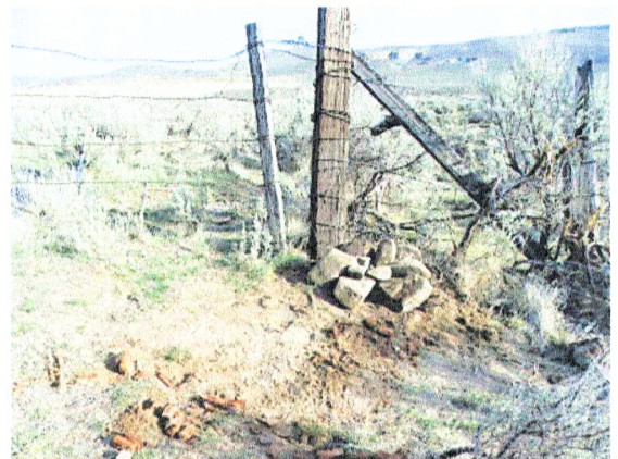
Notice the rotted remains of the original fence post I found buried deep in the ground and where I set the Brass Cap monument. The stone mound is as it appeared before I buried it with soil to help stabilize the stones for the future.
