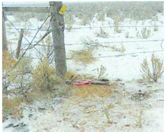
Buried monument to within 3 inches of the surface. Original stone was placed below the surface on the West side of the Brass Cap. No other stone was available in the area; therefore the monument stands alone. I left the original iron pipe I had found lying beside the new monument.
