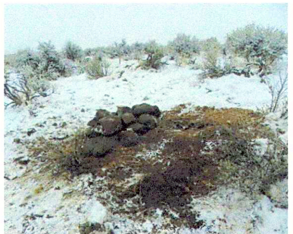
Brass cap and mound of stone as they appeared before covering the mound with soil to assist in protecting and stabilizing the mound. Notice the reference pin located in the background near the top just left of the center of photo.
