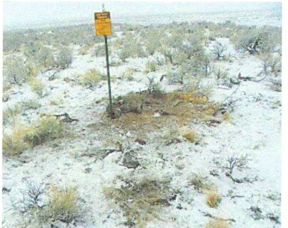
Brass cap and small mound of stone as they appeared before covering the mound with soil to assist in protecting and stabilizing the mound. I then reset the steel fence post reattaching the monument sign to aid in locating the monument in the future.
