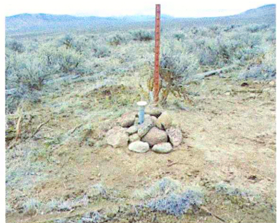
Brass cap and mound of stone as they appeared before covering the mound with soil to assist in protecting and stabilizing the mound. I then reset the steel fence post alongside the mound to aid in locating the monument.
